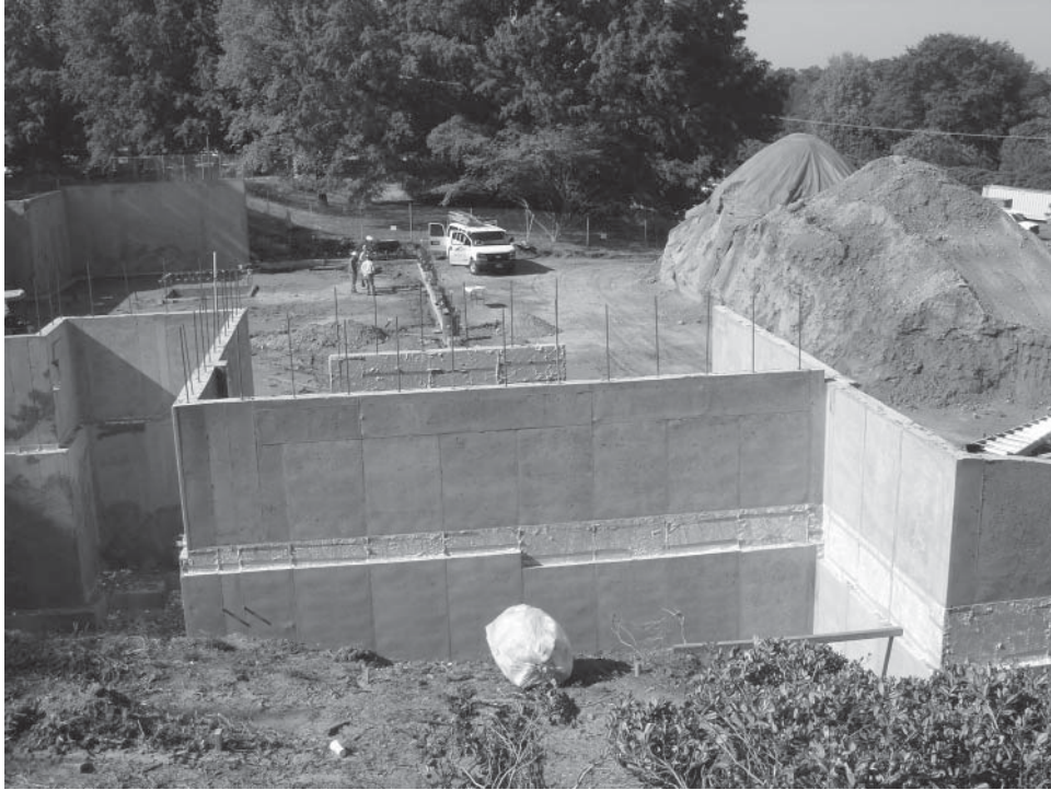
Retaining wall with stepped wall thickness.
