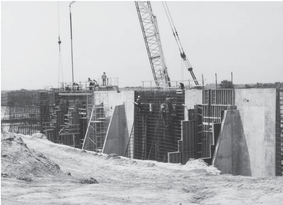
Thirty-two-foot-tall foundation walls for the MCI Mid-Continent Data Center in Omaha, Nebraska.
