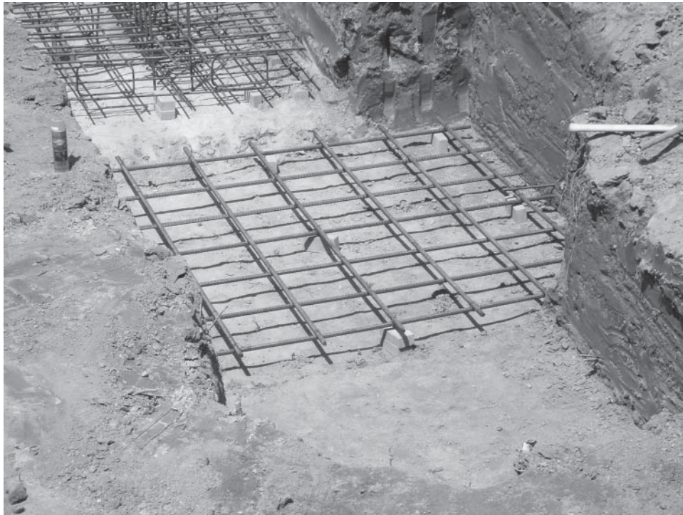
Single column footing prior to placement of column reinforcing.
