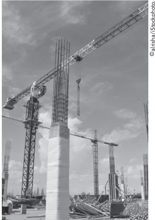
Reinforced concrete columns.
