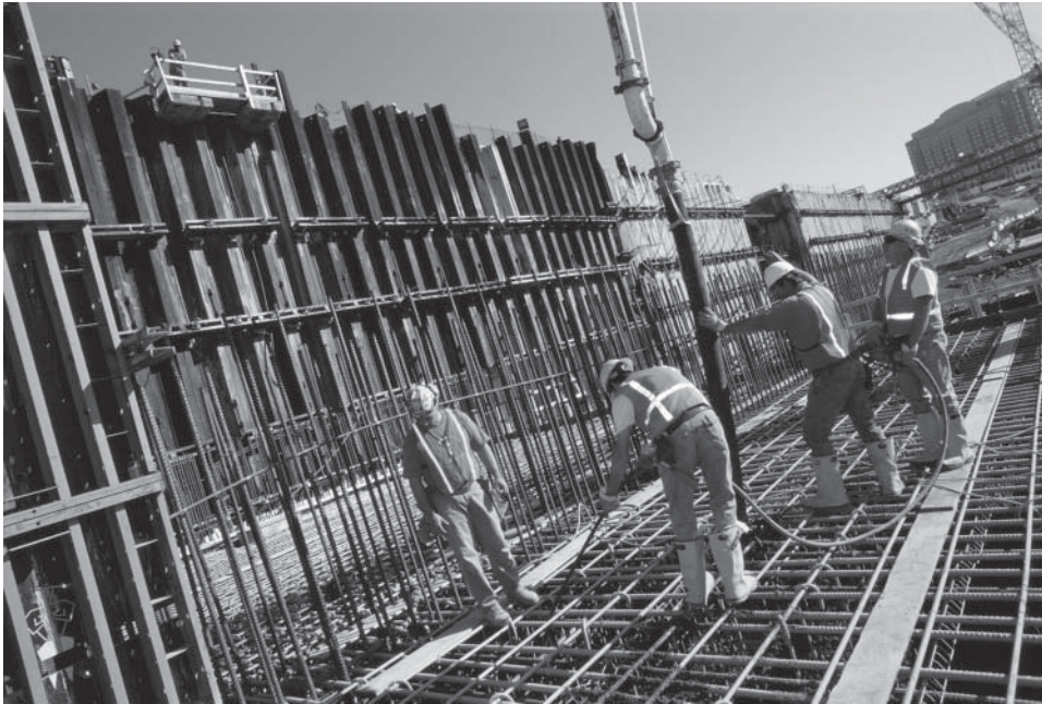
Pouring concrete, Big Dig, Boston, Massachusetts.
