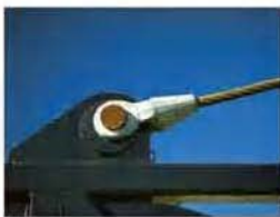
The cable exerts a force on the bracket in the direction of the cable. (1)
