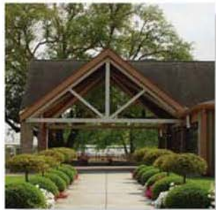
The forces in the members of this simple roof truss can be determined using the method of joints.
