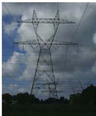
For economic reasons, large electrical transmission towers are often constructed using space trusses.
