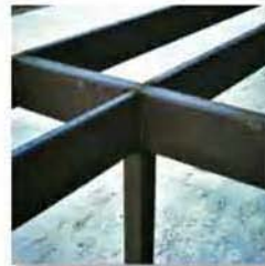
The floor beams of this building are welded together and thus form fixed connections. (10)
