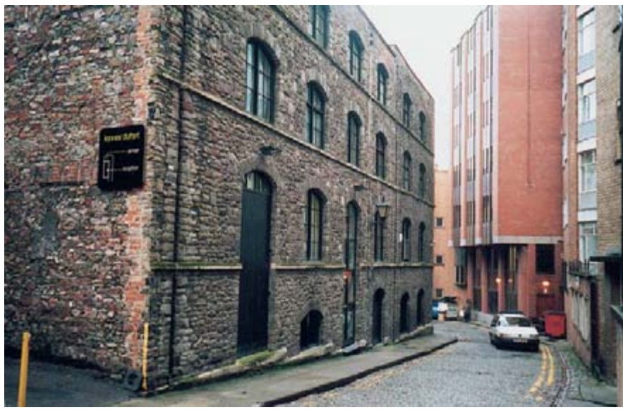
The exterior of the building
