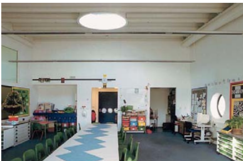
View of a classroom towards the rear, showing the effect of the daylighting and the circular rooflight.
