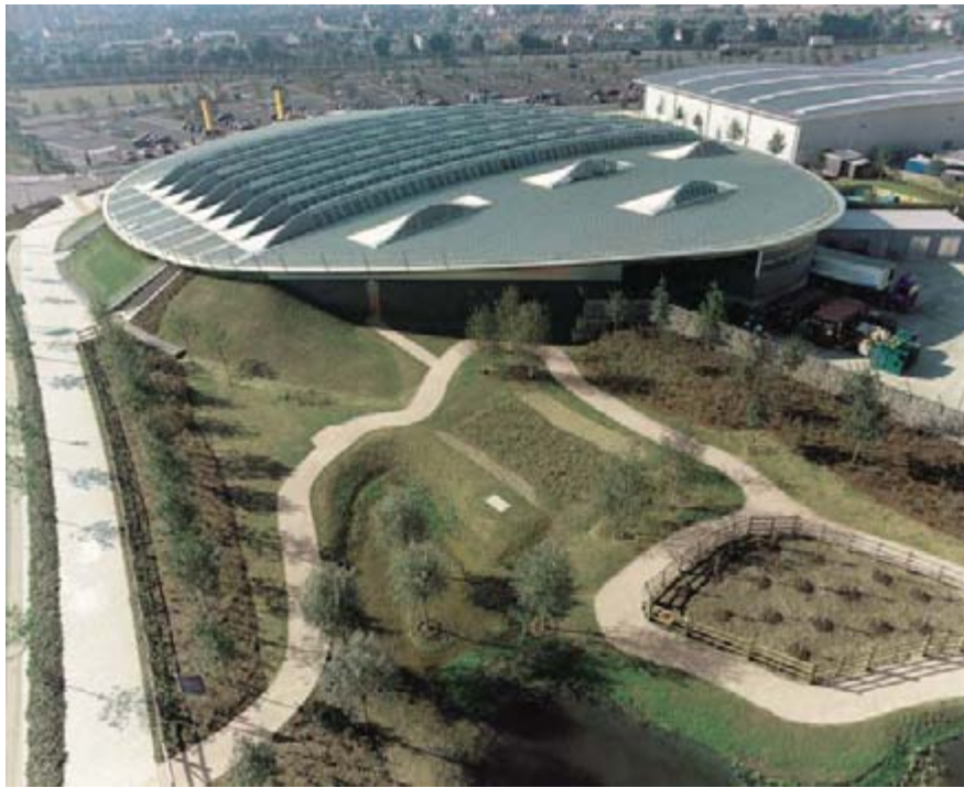
The roof from above
