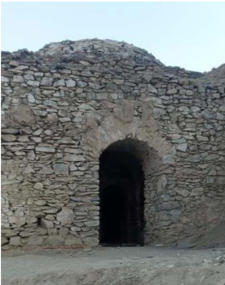
A picture of a Buddhist temple after renovation
