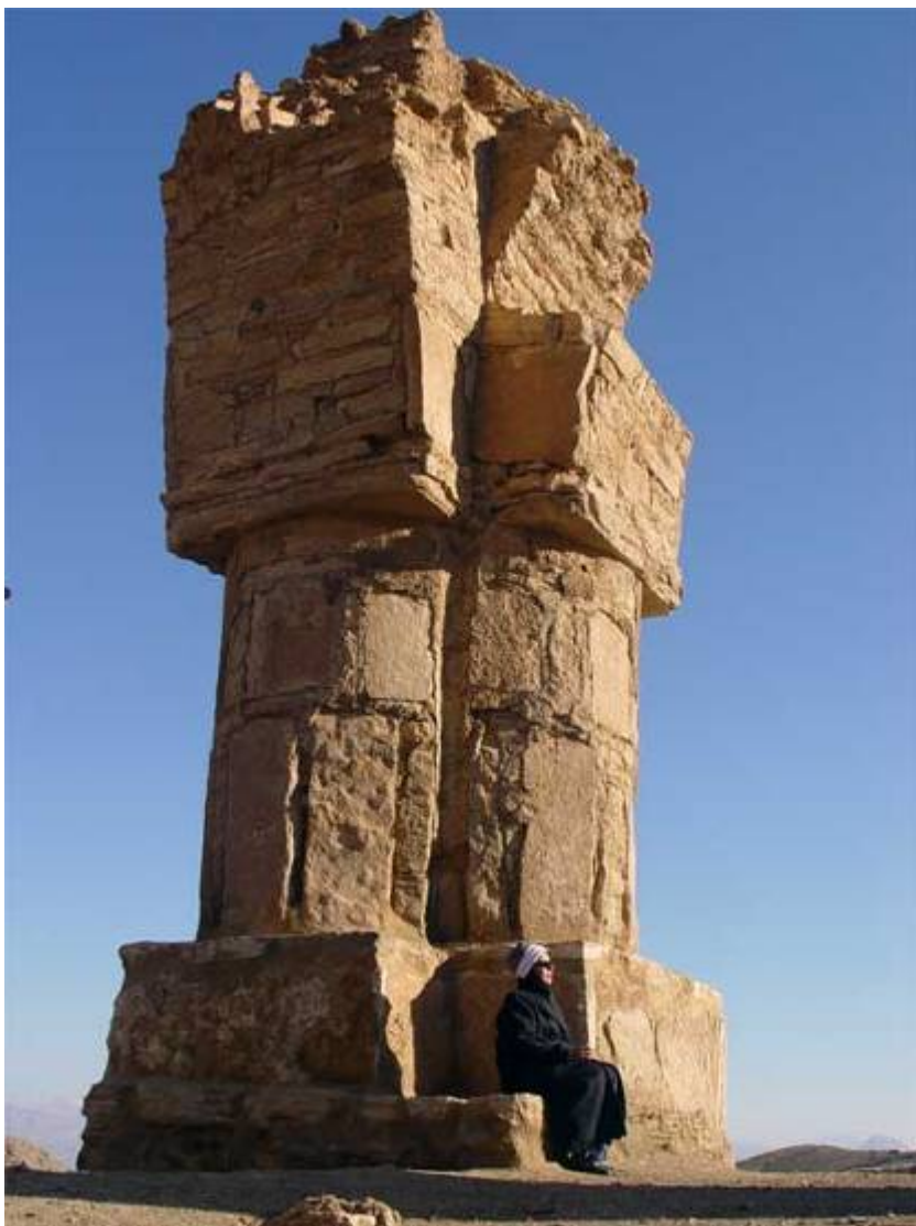
Figure 4.2: Botkhaneh Tetrapylon, the northeastern pillar
