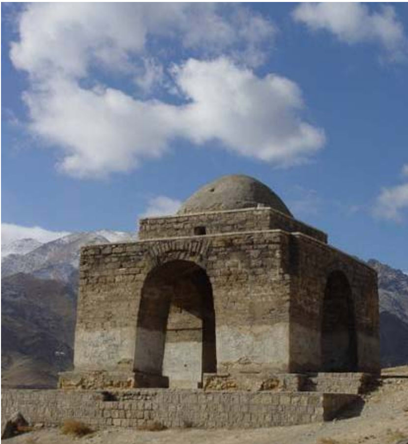
Figure 3.1: Niasar Tetrapylon, the western view
