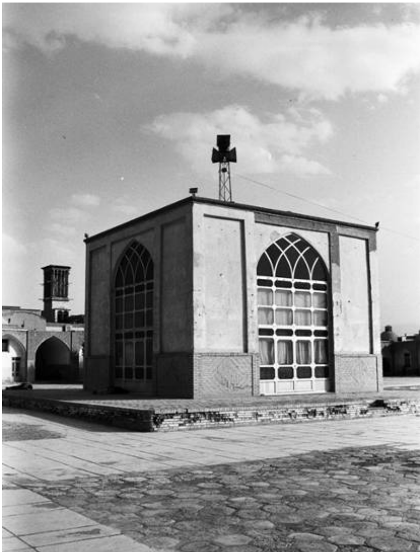
Figure 11.8: Mosalla Tetrapylon, Yazd
