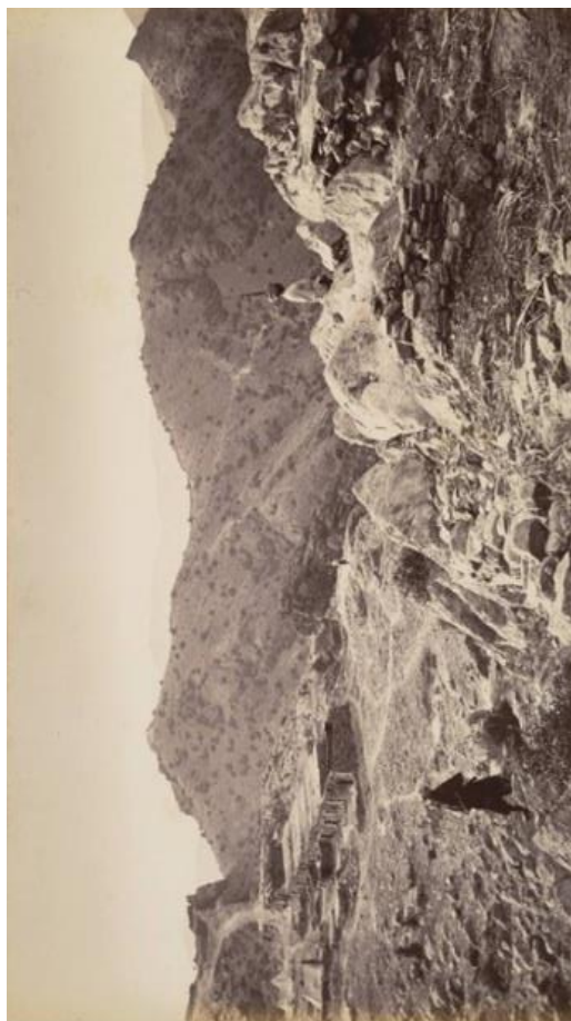
Photograph taken by John Burke in 1878, with the view looking up the western wall of the Ali Masjid fort in the Khyber Pass, showing the right corner bastion & position of the three conical peaks forming the Afghan forces' right defence, with an line of sangar. The sangar were defensive stone breastworks.
