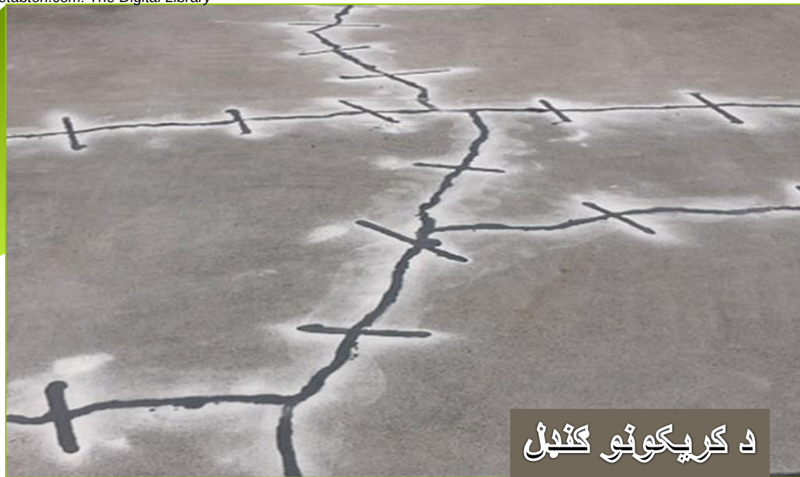
Figure 3: Stitching & Doweling
